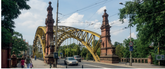
Zwierzyński Bridge, photo from the WPM UMW collections
